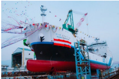
Launching "SUIISO FRONTIER" in Kobe
